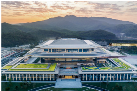
Baiyun International Conference Center Phase II
