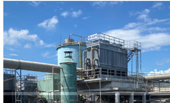
Closed cooling tower transformed by Guangzhou Paper has successfully solved the problem of sewage odor diffusion
